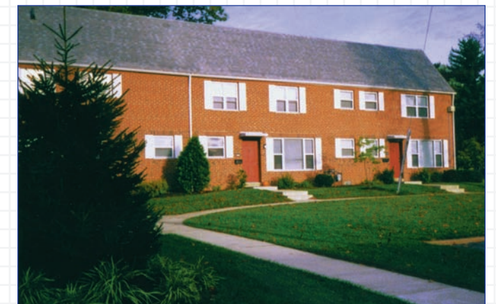
A close-up of one of the 56 buildings located on the property.
