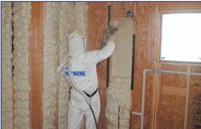
*Icynene was so effective as an air barrier that Mr. Knight won permission from local building inspectors to reduce ceiling insulation to a total of R-19, far below what codes typically require.*
